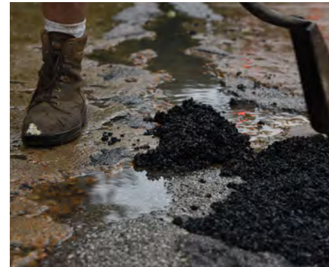
EZ Street asphalt works in water filled potholes
